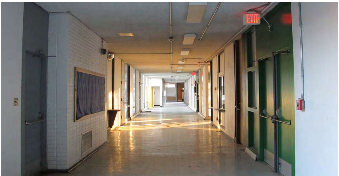
Photo of St. Francis Xavier School hallway - the light at the end of the tunnel.
